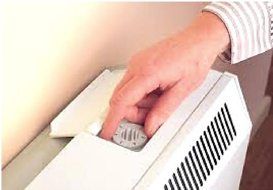
Avoid using the convector button (boost), if there is one. It is better to turn up the input on your storage heater and store more heat. Understanding how to operate your storage heaters as effectively as possible will help you to stay warm enough and not waste energy.
